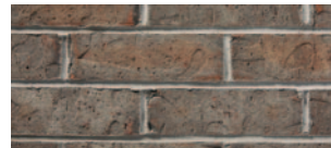
CONCAVE | MORTAR JOINT
