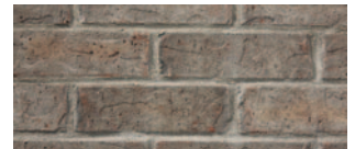
RAKED | MORTAR JOINT
