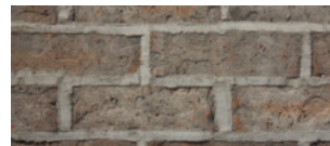
FLUSH TROWELED | MORTAR JOINT
