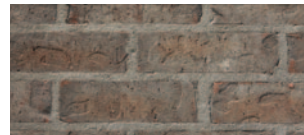
FLUSH BRUSHED | MORTAR JOINT
