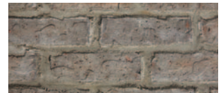
OVERGROUT | MORTAR JOINT
